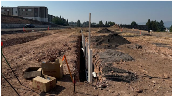
Under slab rough-in plumbing has been completed.
