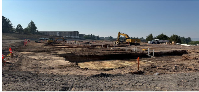
View of foundation work happening.
