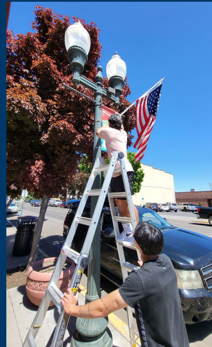
Main Street Flags Installation
